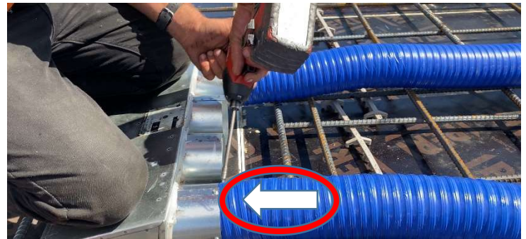
Figure 2 : Use self-drilling screws to mechanically fasten the duct
