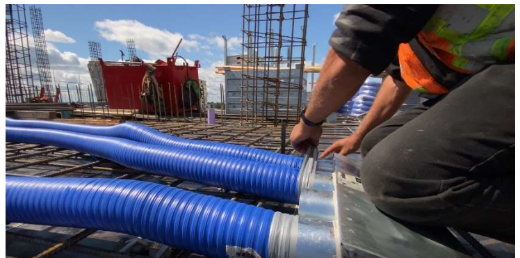
Figure 3: Add a layer of FLEXTAPE
