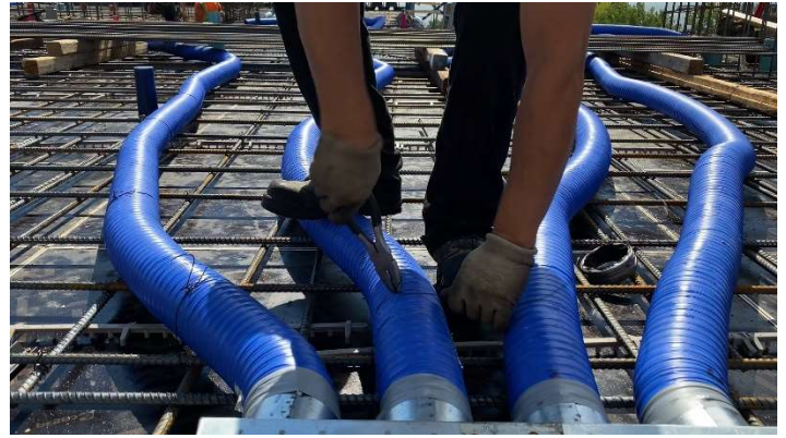
Figure 4 : Firmly fix the FLIXS duct to the reinforcement at regular intervals of 30 cm
