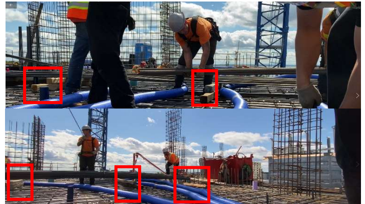
Figure 6 : Double the wooden supports when rebars are placed on the FLIXS
