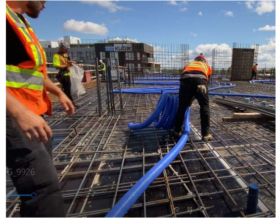
Figure 1 : Unroll the duct to the required length following it's direction.
