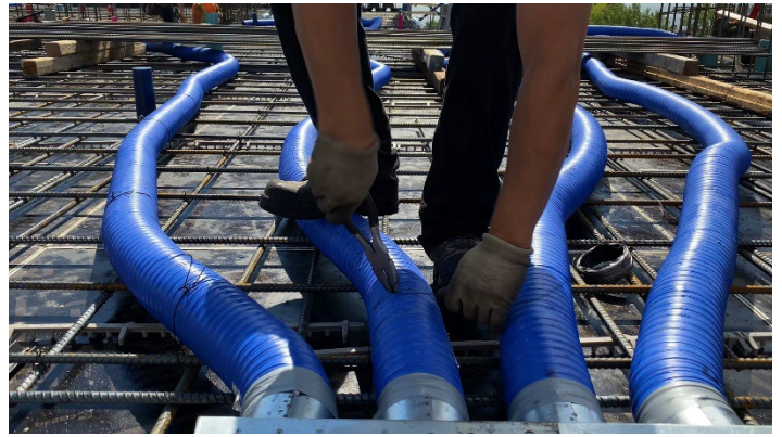
Figure 4: Securely fix the FLIXS to the frame at regular intervals of 30 cm.
