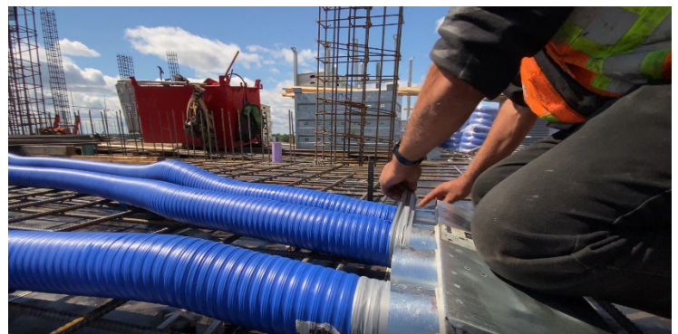
Figure 3: Add a layer of FLEXTAPE tape.
