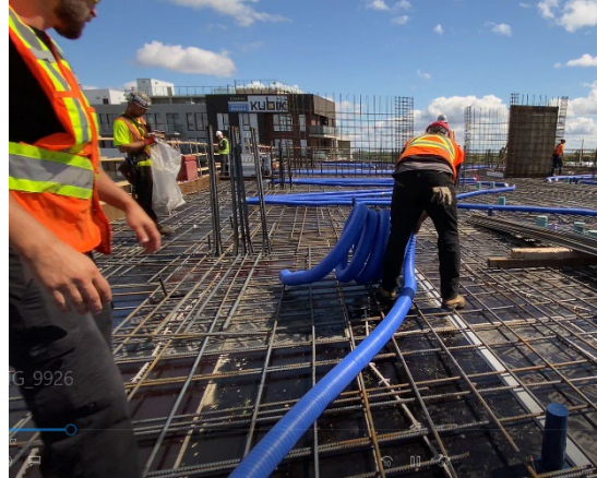
Figure 1 : Unroll the flexible air duct to the required length following the direction of the air flow.
